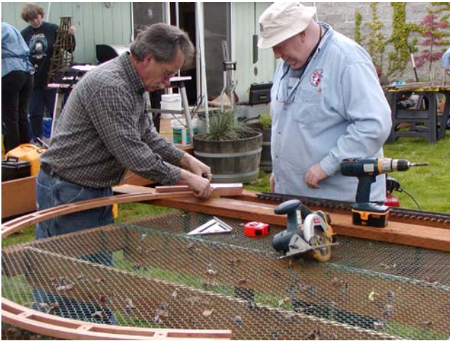
Gary Lee and Nick Kelsey prepare a turn-around roadbed which will be supported by one of the tall trestles.
