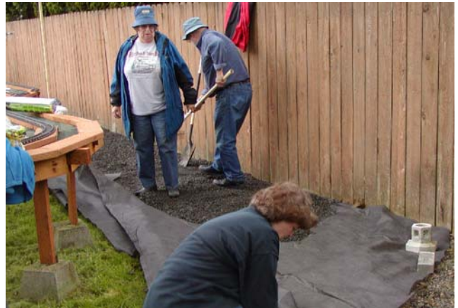
Penny Walker, Bud Quinn, and Sue Kelsey install ground fabric and gravel for the gravel path. Not shown is Larry Blair moving a heroic load of gravel from the dump to the site.
