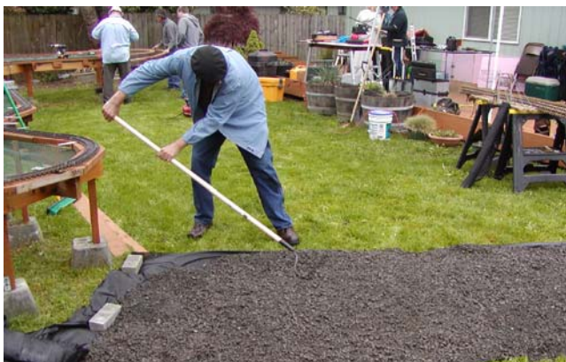
Jerry Clark levels and smooths the gravel path
