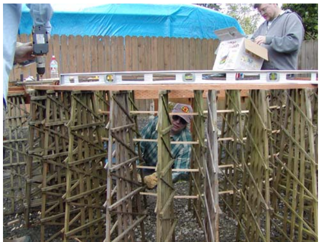
Jan Zweerts literally climbs into the work as the second trestle is installed
